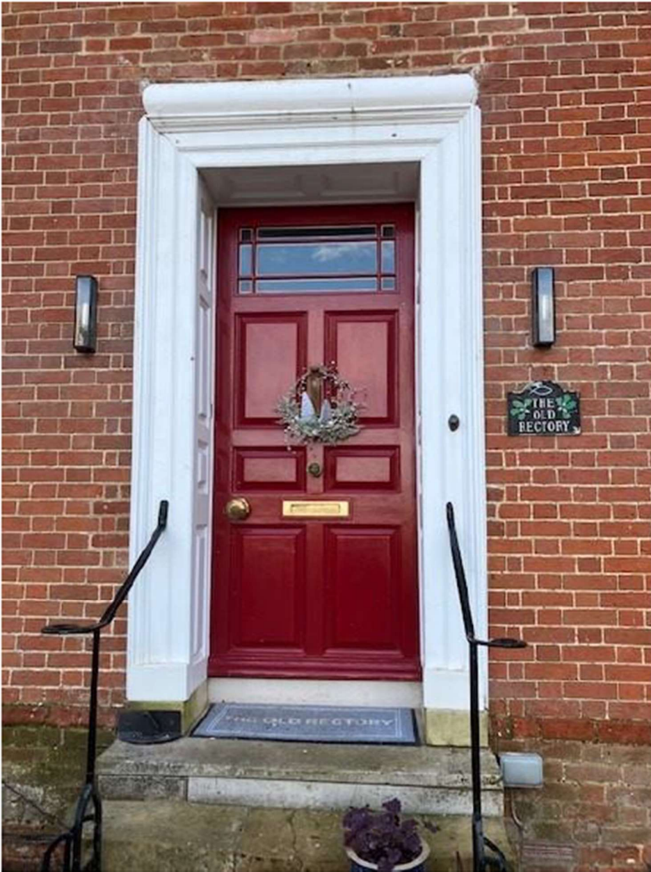
Existing doorway with pediment removed
